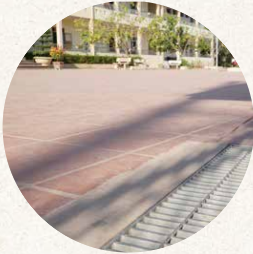
Construction of drainage system in Cam Hai Primary & Secondary school
